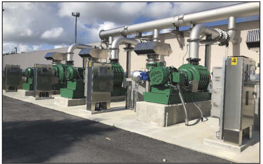
Figure 5. New Multistage Centrifugal Blowers at the Regional Wastewater Treatment Plant
