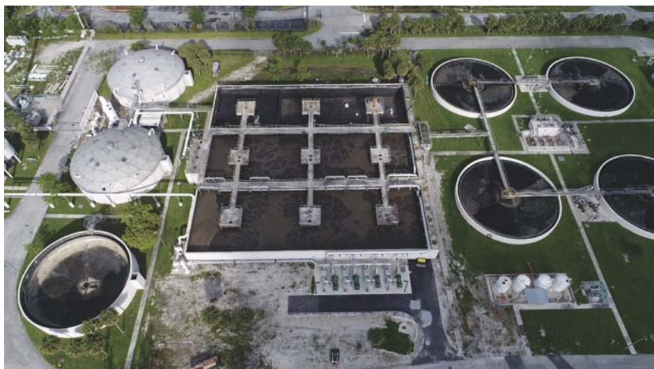
Figure 1. Plantation Regional Wastewater Treatment Plant
