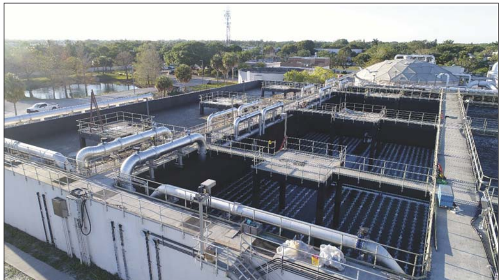
Figure 6. New Fine Bubble Diffused Aeration System at the Regional Wastewater Treatment Plant
