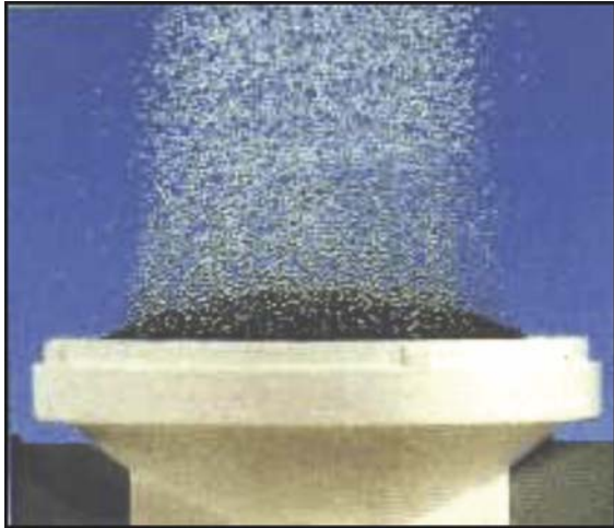
Figure 4. Fine Bubble Diffuser (photo: ITT Water and Wastewater – Sanitaire)
